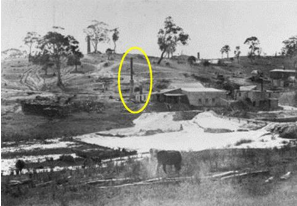
FIGURE 10-34 | VIEW OF CHIMNEY AND TAILINGS DAM FROM OTHER SIDE OF THE VALLEY, C1887
