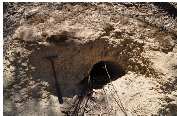
FIGURE 14-10 | LOCATION 3, RABBIT BURROW IN BIH TAILINGS DAM.
