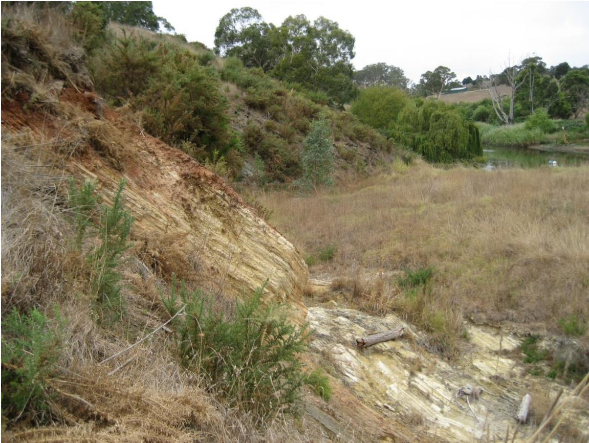
FIGURE 14-20 | LOCATION 8 - EXPOSED TAILINGS AT NEW ERA, PHOTOGRAPHED BY MAXIMUS, MARCH 2007
