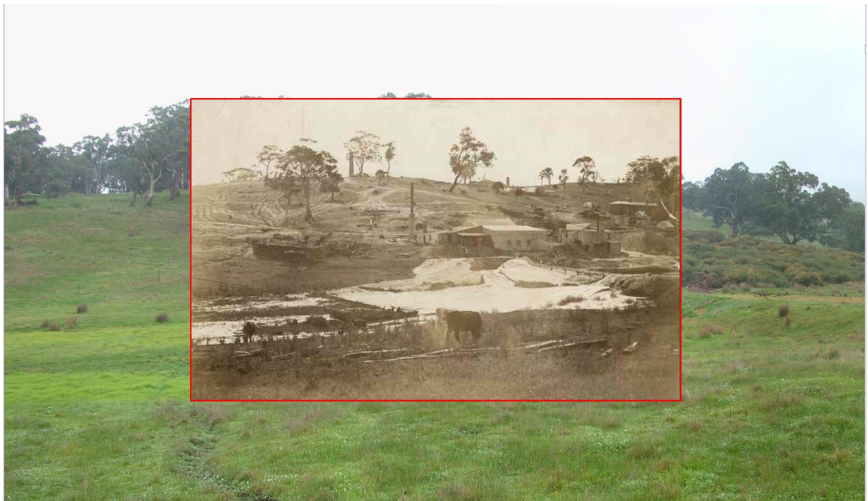
FIGURE 14-13 | LOCATION 6, CENTRAL PHOTOGRAPH SHOWS RIDGE TAILINGS DAM OVERFLOWING C1880, DPC PHOTOGRAPH B6260
