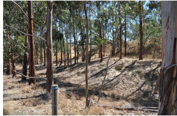
FIGURE 14-9 | LOCATION 3, - WESTERN LIMIT OF BIH TAILINGS DAM IS LOCATED ON PROPOSED OPERATING SITE.
