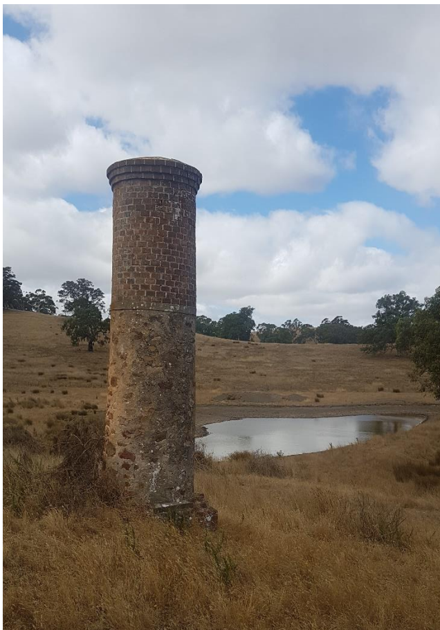
FIGURE 17-8 | RIDGE MINE'S TAILINGS DAM AND CHIMNEY. FACING SOUTH.
