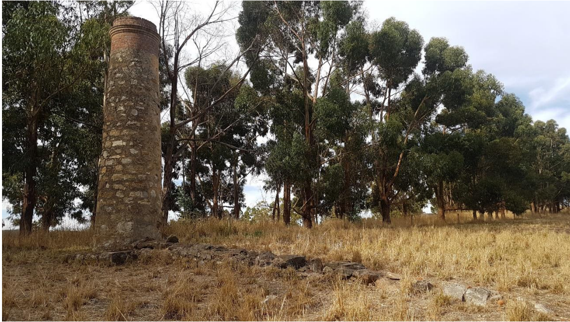
FIGURE 17-7 | LONE HAND CHIMNEY AND FLUE. FACING EAST.
