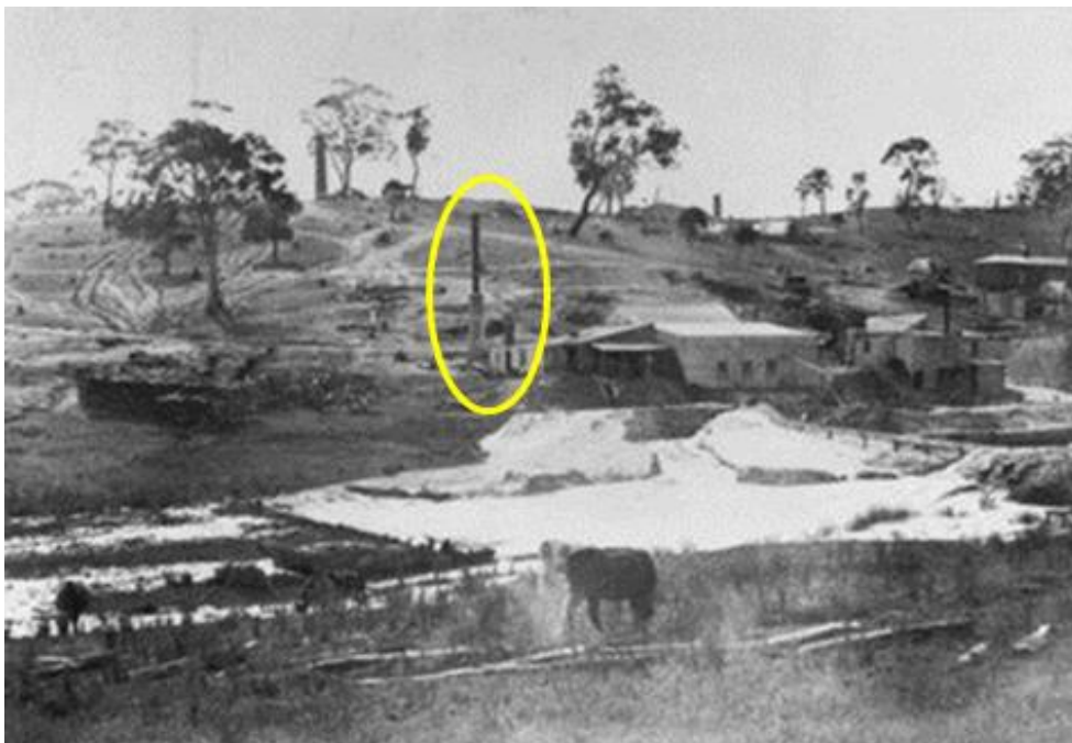
Figure 22-8 | View of chimney and tailings dam from other side of the valley, C1887
