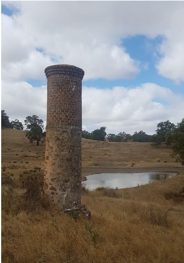
Figure 22-7 | Ridge Mine's tailings dam and chimney. Facing south.
