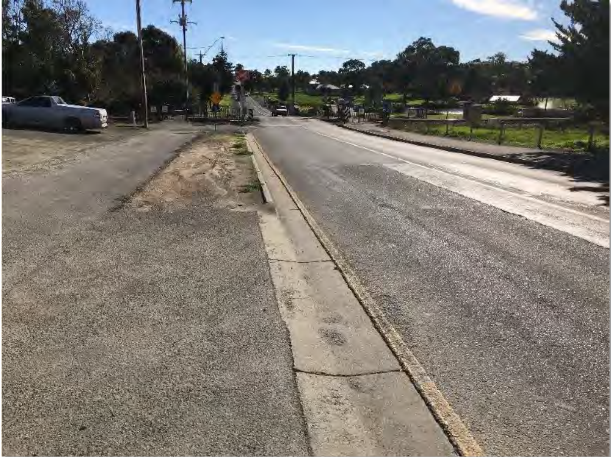
FIGURE 3-106 | UPGRADES TO THE RAIL CROSSING AT NAIRNE ARE RECOMMENDED TO IMPROVE SAFETY FOR ALL USERS. (IMAGE LOOKING NORTH, APPENDIX F1)
