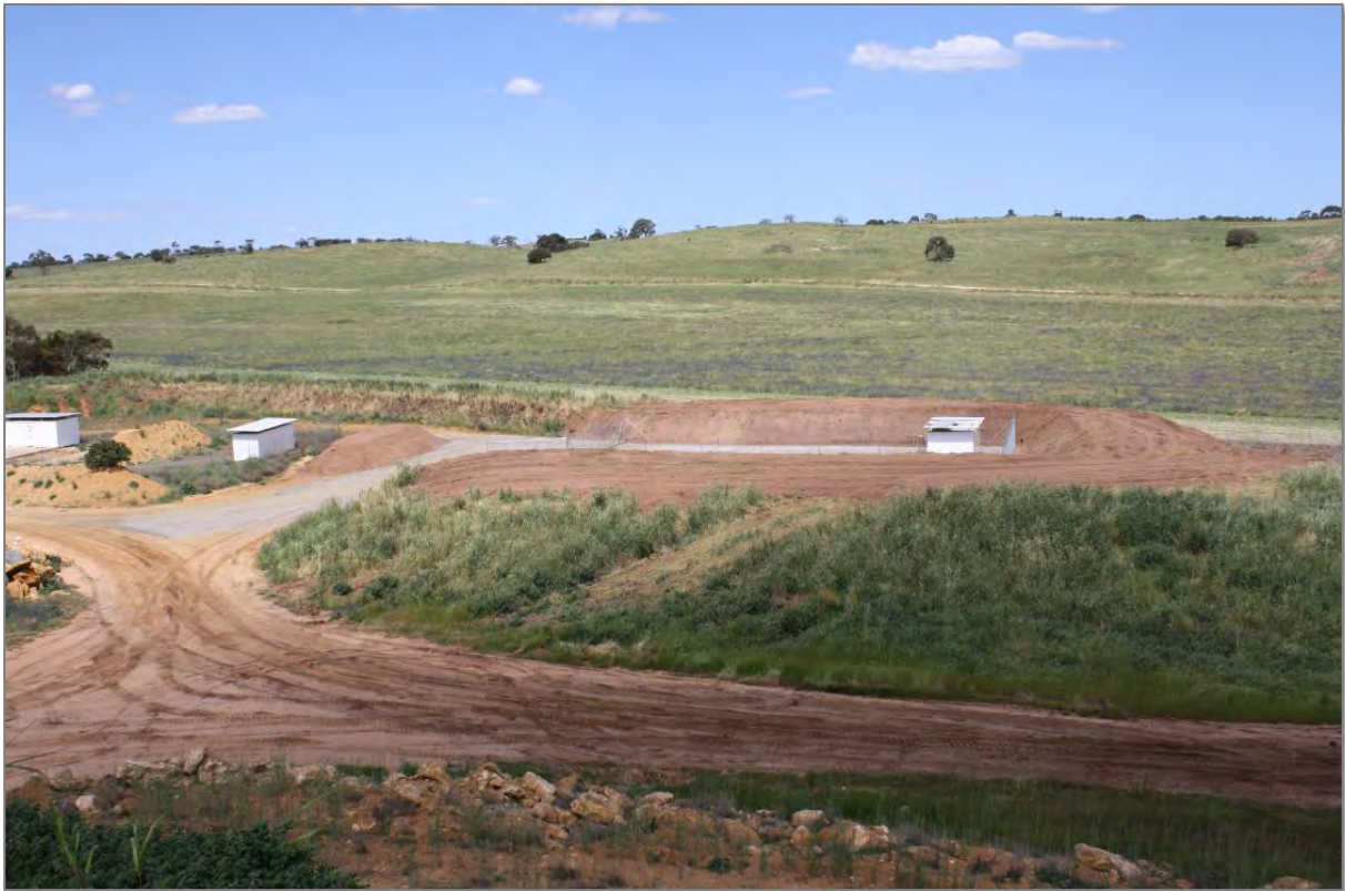
FIGURE 3-81 | VIEW OF THE EXISTING LICENCED MAGAZINE COMPOUNDS AT AZM
