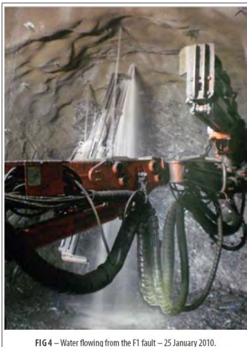
FIGURE 3-61 | EXAMPLE OF GROUNDWATER INFLOW EXPERIENCED AT ERNEST HENRY MINE, 2010, WHICH WAS MANAGED THROUGH A GROUTING PROGRAM
