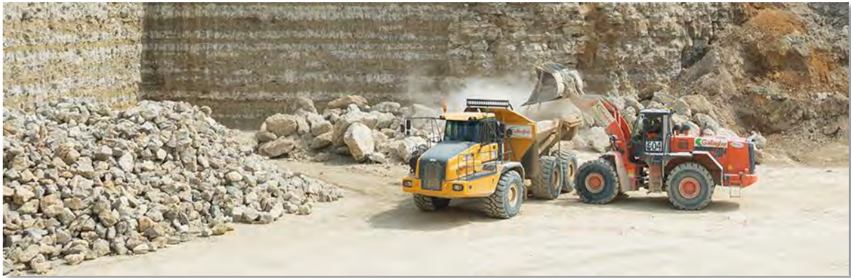
FIGURE 3-102 | TYPICAL EQUIPMENT ON SITE FOR IML, BACKFILL LOADING (GALLAGHER, 2017)
