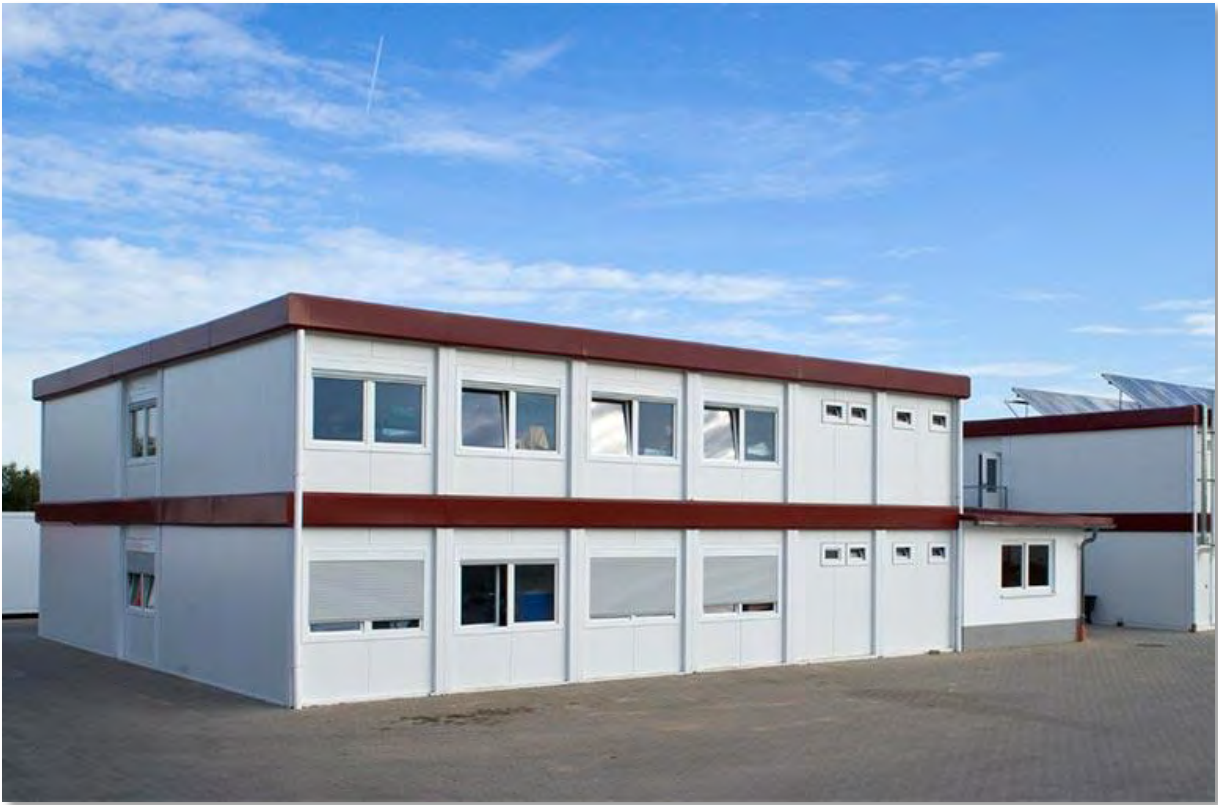
FIGURE 3-145 | TYPICAL MODULAR OFFICE LAYOUT PROPOSED FOR THE BIH SITE. (LOSBERGER DE BOER GROUP, 2017)
