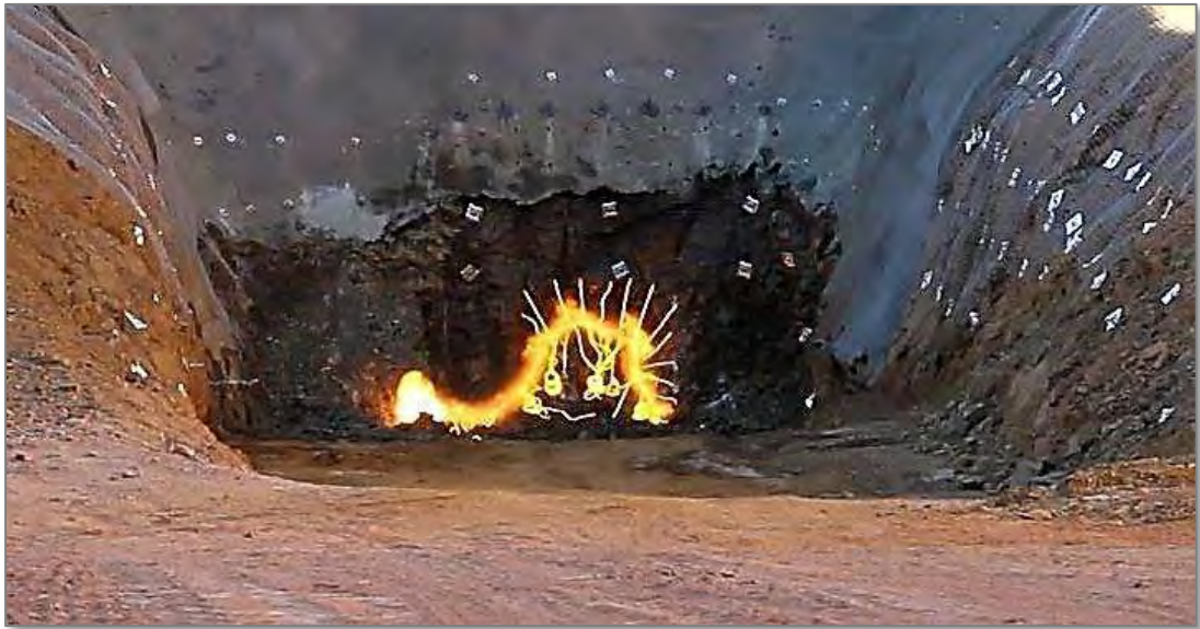
FIGURE 3-82 | FIRING OF INITIAL DECLINE CUT IN A BOXCUT (AMPT SERVICES, 2017)
