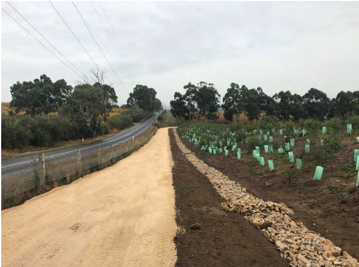
FIGURE 3-152 | NEWLY CONSTRUCTED STORMWATER CONTROL BUND WITH INFILL VEGETATION AND EROSION CONTROL ALONG BIRD-IN-HAND RD (2016)
