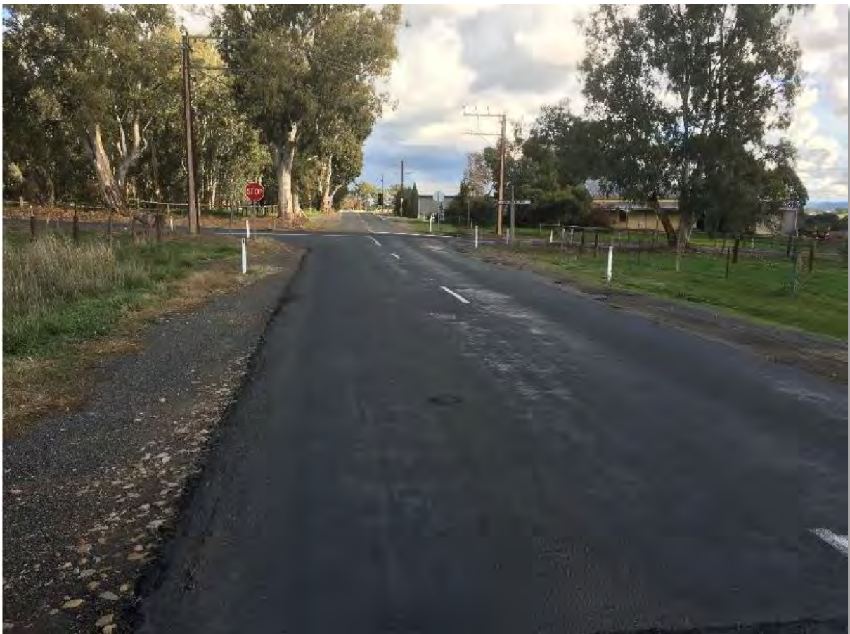
FIGURE 3-105 | PFEIFFER ROAD/NAIRNE ROAD INTERSECTION LOOKING WEST FROM PFEIFFER RD (APPENDIX F1)
