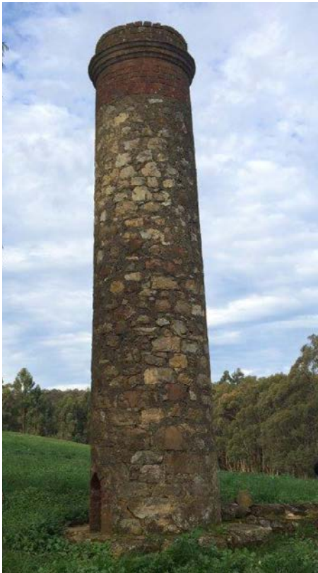
State Heritage Listed Chimney + Flue (Lone Hand Site)
