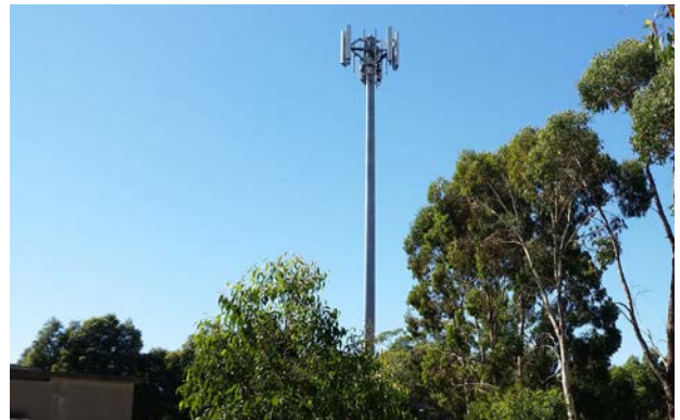
Mobile phones towers (Ridge Road)
